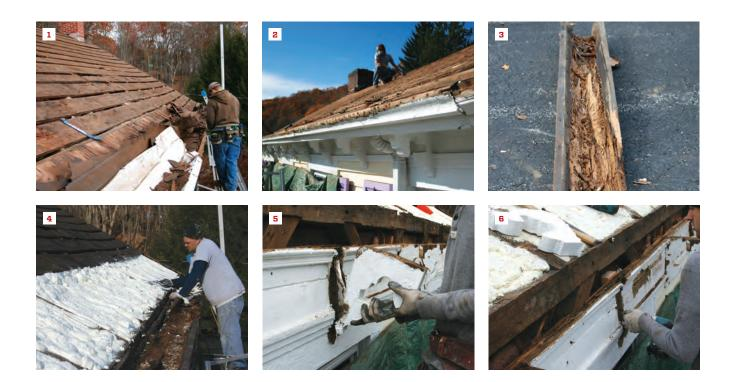
that the original wood trough had deteriorated; where the gutter was sagging the most, it was cracked and severely rotted (2). The gutter was big—8 inches deep, 12 inches wide, and 39 feet long—so we cut it into manageable pieces with a chain saw to safely get it to the ground (3).
