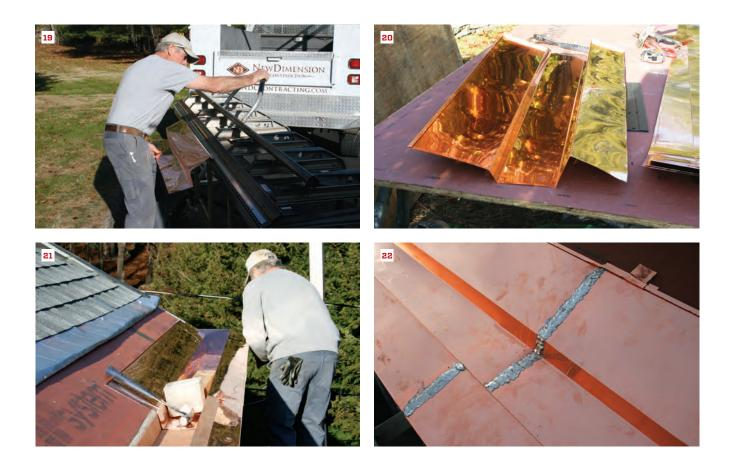
the drip edge and settled the panel into the trough (21), then secured it on the roof side with 1½-inch-wide copper cleats 24 inches on-center, fastened to the sheathing with 1½-inch-long copper nails. We overlapped the next liner panel by 3 inches, then soldered the seam (22) (see Soldering Seams, facing page). With two panels in place at one end, we switched sides and installed two panels at the other end.
