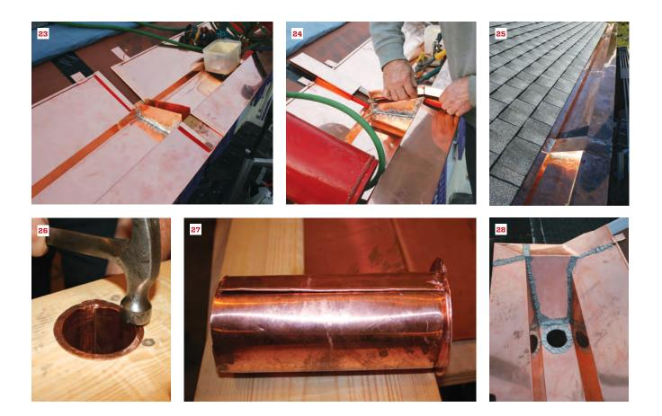
met the trough, we bent a ½-inch leg that would form the soldered connection. To install these pieces, we slipped the legs under the liner trough, molded the upper portion to the roof, the crown-mold-ing cap, and the gutter return, and soldered the seams (28).
